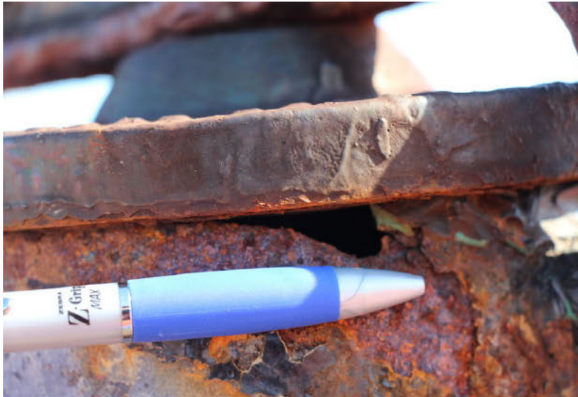
Figure 11: Closer view of the area pictured in Figure 10. Picture taken by the U.S. Coast Guard on November 6, 2017.
