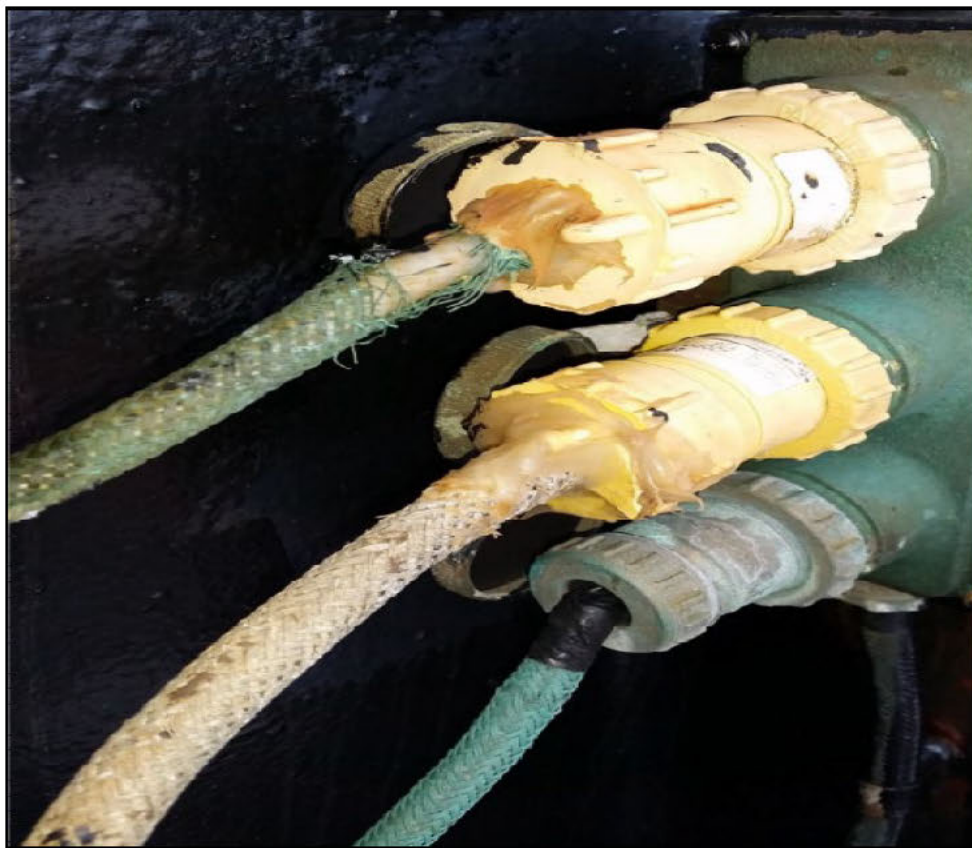
Figure 18: Exposed forward mast plugs located on the forward section of the barge. Picture provided by ABS.
