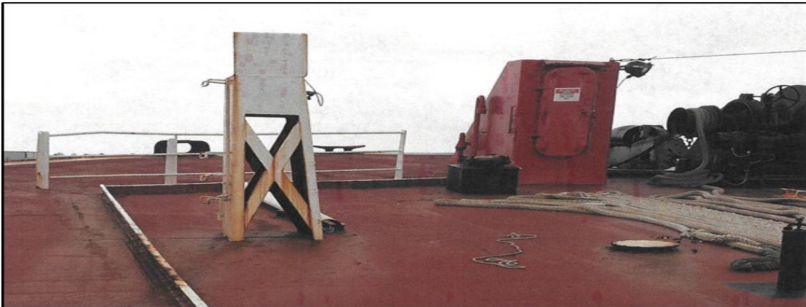
Figure 3: Picture of the "doghouse", which provides access to compartment 2 of the forepeak, located on the bow of B. NO. 255. The anchor windlass is located on the right side of the doghouse in the picture. Picture provided by ABS.
