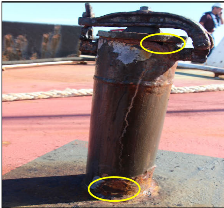
Figure 10: Picture of the number one starboard cargo tank ullage tube leading directly to the cargo tank on B. NO. 255. Circles added. Picture taken by the U.S. Coast Guard on November 6, 2017.
