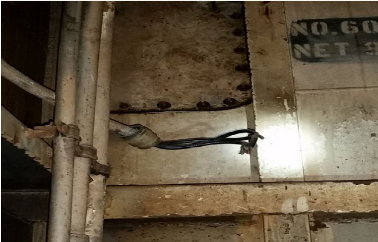
Figure 17: Dead-end wires in forward rake. Picture provided by ABS.
