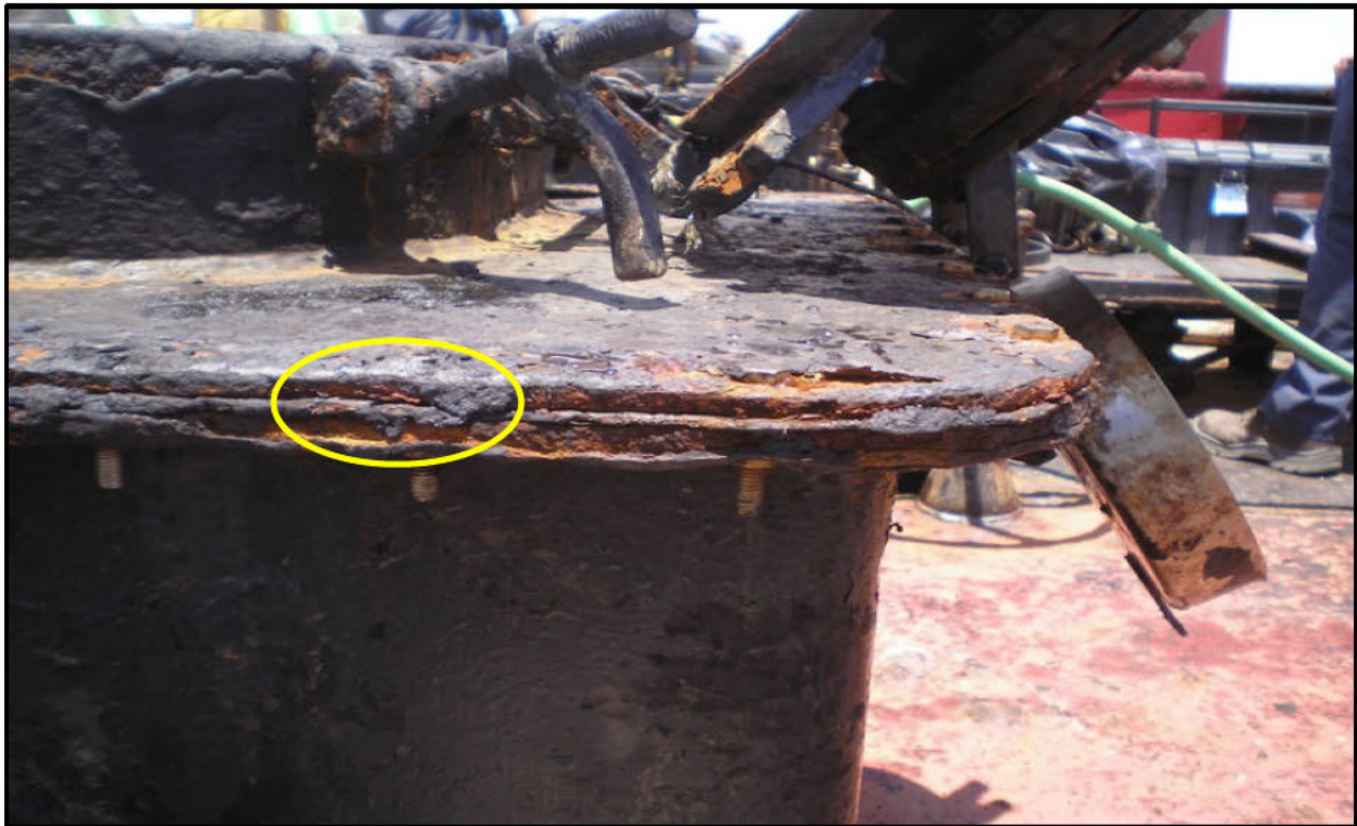
Figure 14: Picture of wasted cargo tank hatch on B. NO. 255. Circle added. Picture taken by the U.S. Coast Guard in June 2018.
