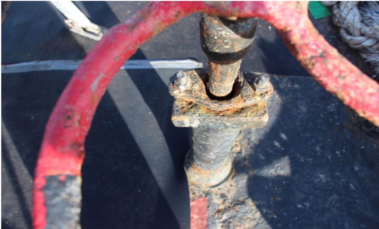
Figure 21: Picture of the number one starboard cargo tank main valve stem on the B. NO. 255. Picture taken by the U.S. Coast Guard on December 12, 2017
